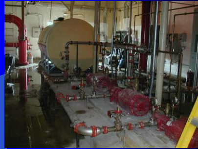
Typical ILBP Pump Skid Installation
