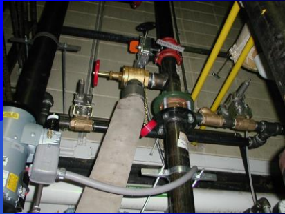
Riser isolation and test outlet valve
