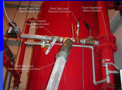
Pressure transducers measure foam concentrate and water pressures
