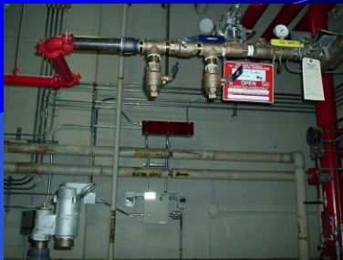
ILBP Foam Risers Fitted with Future Connections for Use with Planit Safe Interface Tank
