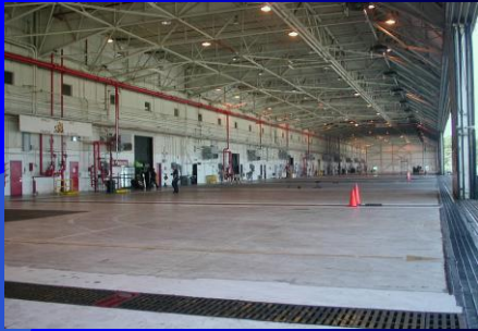
Typical Navy ILBP Foam Stations Hangar Installation
