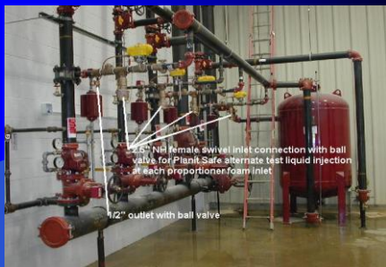
Planit Safe connections on bladder tank system with multiple risers
