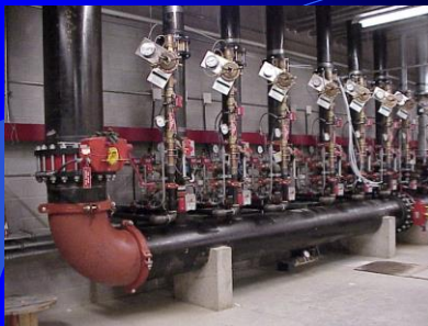
Planit Safe Test Setup to Measure Flow and Injection Rate of 8 Risers Operating Simultaneously
