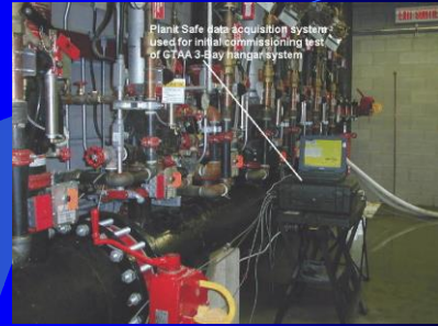
Planit Safe Test Setup to Measure Flow and Injection Rate of 8 Risers Operating Simultaneously
