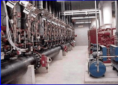
24 ILBP Risers Protecting a 3 Bay Aircraft Hangar Total System Flow 18,000 gpm
