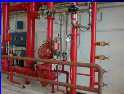
Typical ILBP Navy Foam Riser Fitted with Conductivity Sensor
