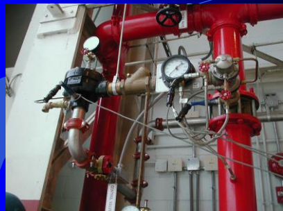
Typical ILBP Navy Foam Riser Fitted with Pressure Transducers
