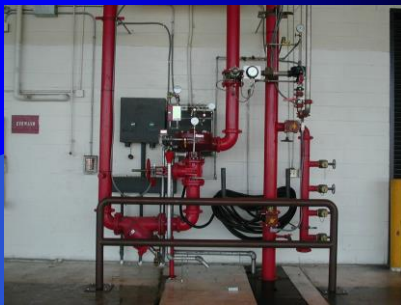
Typical Navy ILBP Foam Riser in Hangar
